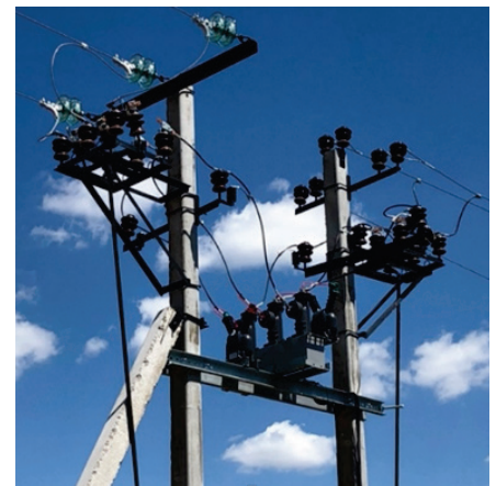
FIGURE 1. Installation example for reclosers, switching module and control unit
