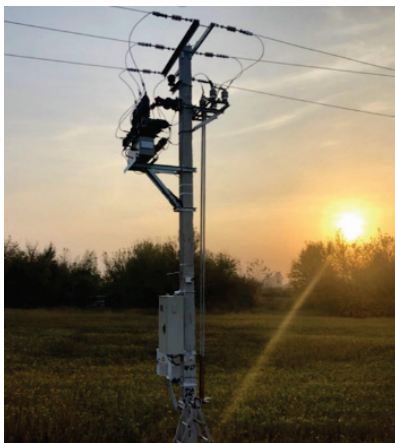
FIGURE 1. Installation example for reclosers, switching module and control unit
