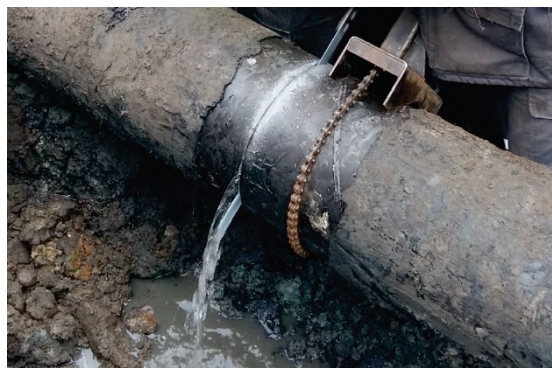
FIGURE 1. Cutting of the DN300 gas pipeline at Myśliwska Street in Kołobrzeg
