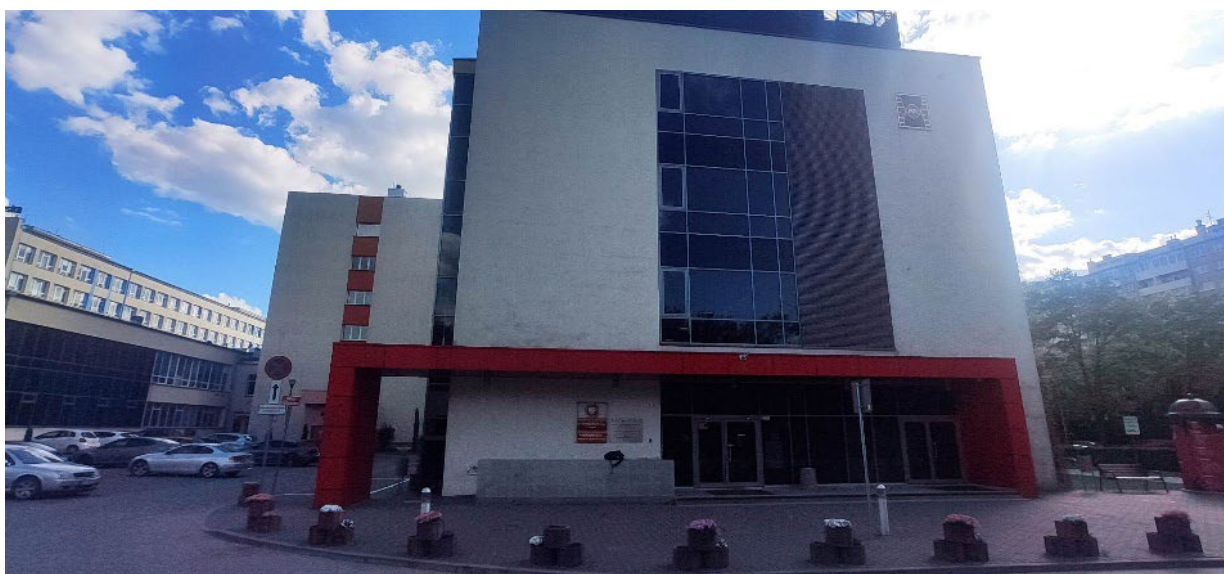
FIGURE 1. Photo of “Energis” from the Northern side – main entrance to the building
