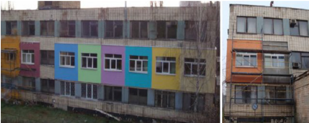
Figure 2. Scheme of insulation of the enclosing structures of the upper floor of building No. 1 of the Institute of Engineering Thermophysics National Academy of Sciences of Ukraine
